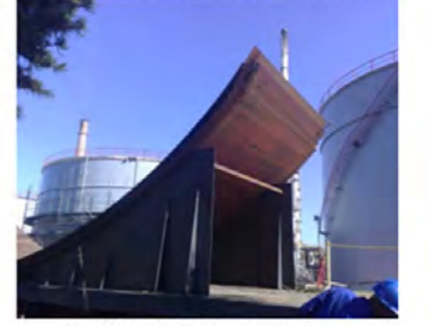
TANK SHELL PLATES
